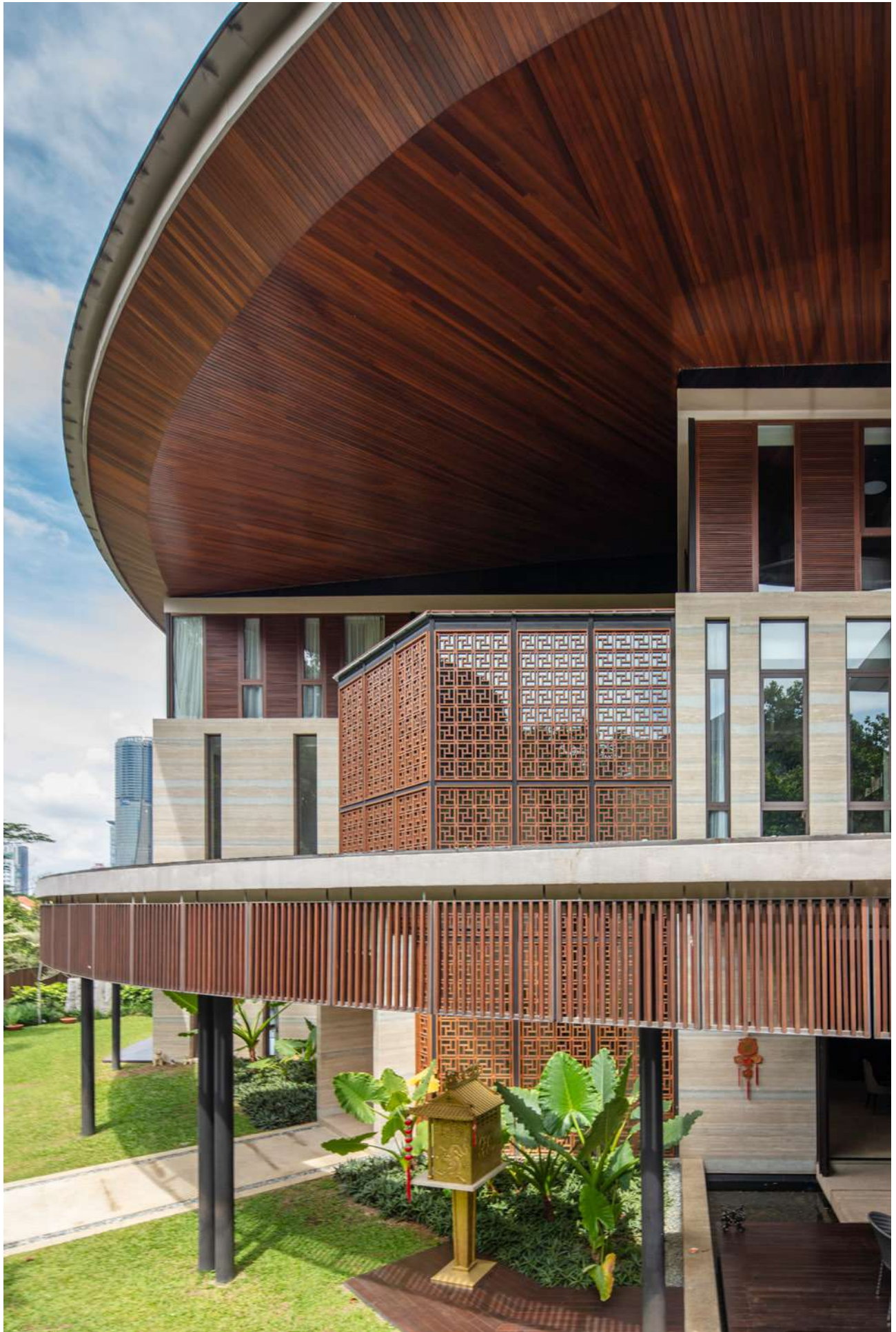
Quadrant House at Seputeh Heights which was designed with an oriental fan shaped roof that provides shelter to the spaces below.
