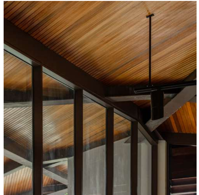
Timber roof truss at the Canopy House.
